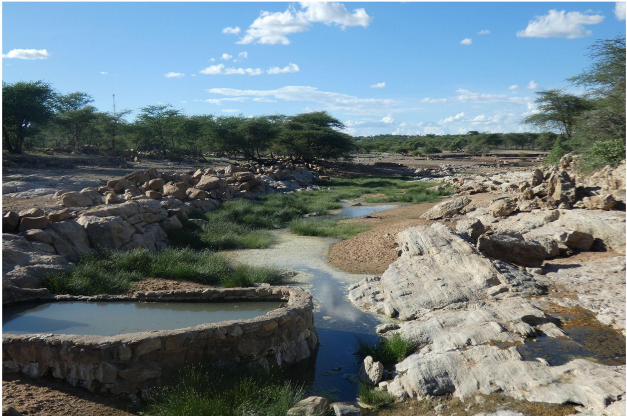
Laisamis Sand Dam, April 2024
